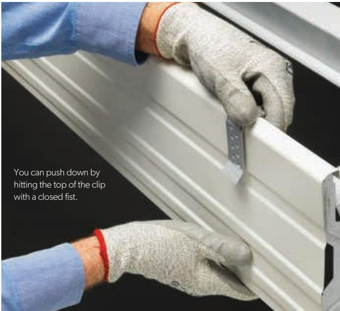
You can push down by hitting the top of the clip with a closed fist.
