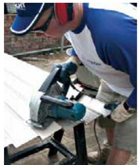
Cut the infill sheets two or three at a time. This equals a single bay and ensures uniformity. Measure twice, cut once.
