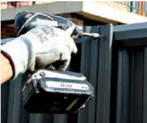
Screw off top rail and make it as close to parallel with the bottom rail as possible. Stand back and look at your work as you go along.
